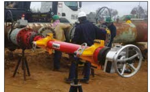
▲ CHT3000 hot tapping application for petrochemical pipeline installation.
