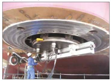
▼ Machining crane bearing face.
